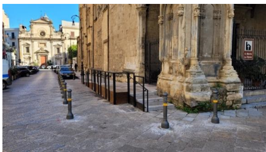
Figure 3. I-Access Project outcomes: Palermo, Church of Santa Maria La Nova: the double access ramp to the churchyard, through the side gate modified for this purpose.
