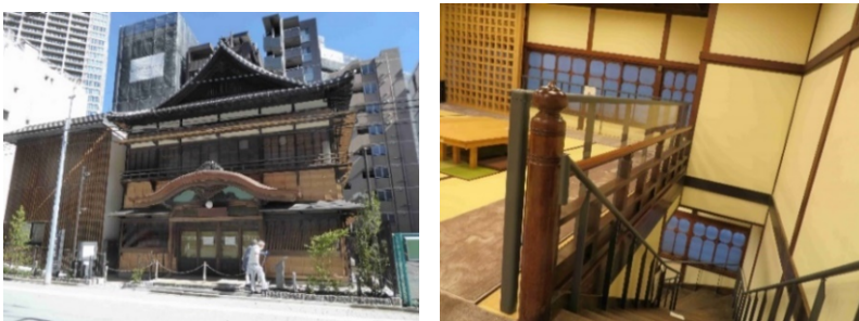
Figure 6a&b. Kenban with elevator annex on the left. Stair guard was added inside.
