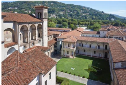
Figure 2. Santa Giulia Monastery, aerial view
