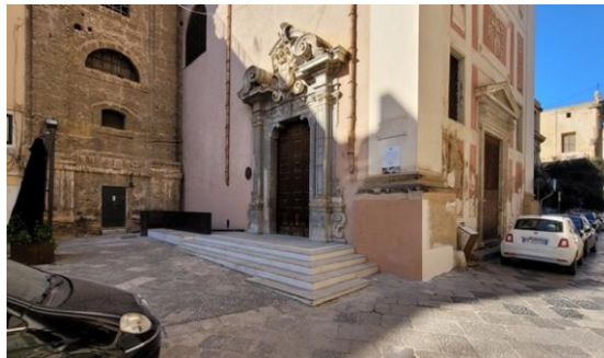
Figure 2. I-Access Project outcomes: Palermo, Church of Santa Maria in Valverde: the ramp for the disabled that engages in the new churchyard, which evokes the original level of the Largo Cavalieri di Malta floor.
