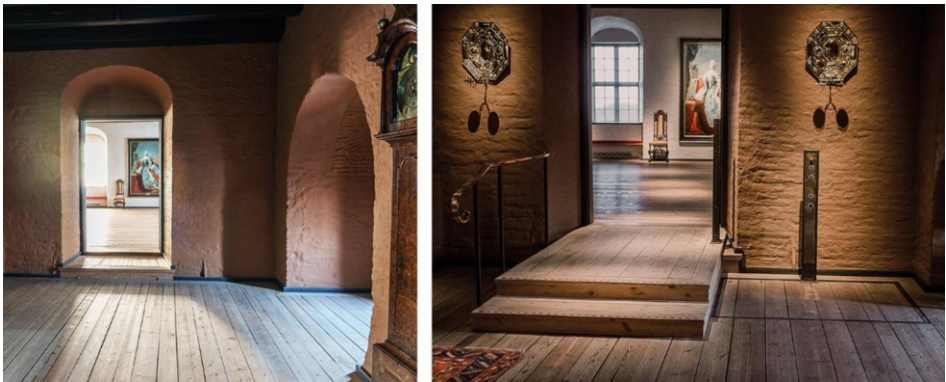
Figure 3. L.h.s.: One of the halls before intervention. R.h.s.: A lifting platform is integrated in the floor. (Photo 1: Oslo Byggentrepreneur AS; 2: A.M. Malkenes Mathiesen/The Norwegian Defense Estates Agency)
