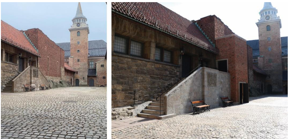
Figure 5. L.h.s.: The courtyard before intervention. R.h.s.: An elevator tower has been established in connection with the new stair. (Photo 1: Arkitektskap AS; 2: M. Brenna)
