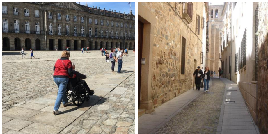
Figure 5: Accessible paving strips in areas of historic paving in Santiago de Compostela and Cáceres.
