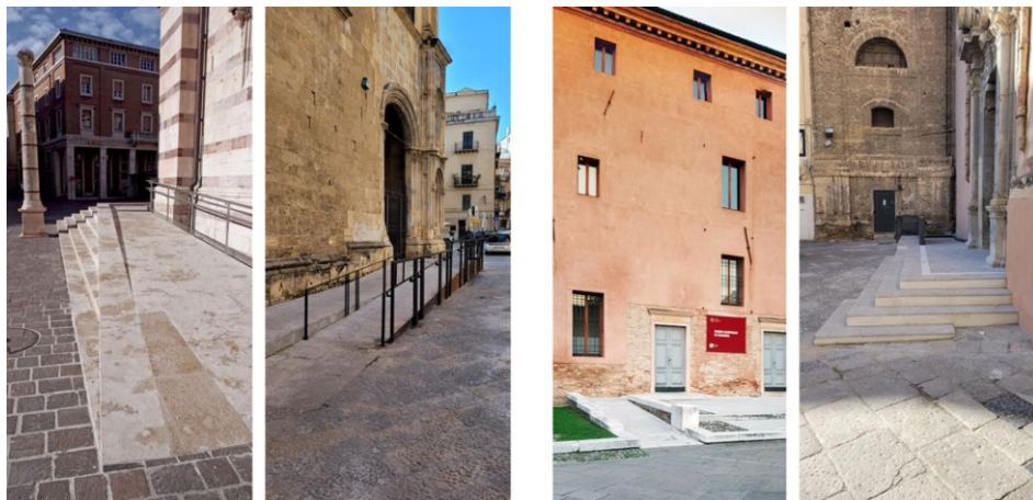
Figure 1. Grosseto, Ravenna and Palermo compared: on the left group, the Cathedral of Grosseto and the disabled access ramp 'landing' in the churchyard, compared to the Church of S. Maria la Nova in Palermo and the construction of the ramp with the same strategy used in Grosseto; on the right group, the National Museum of Ravenna and the new access with the disabled access ramp, compared to the Church of S. Maria in Valverde and the construction of a new churchyard incorporating the disabled access ramp.
